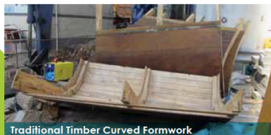
Traditional Timber Curved Formwork
