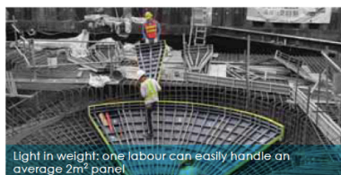
Rapid laying: one semi-skilful labour can assemble 50m 2 formwork per day
